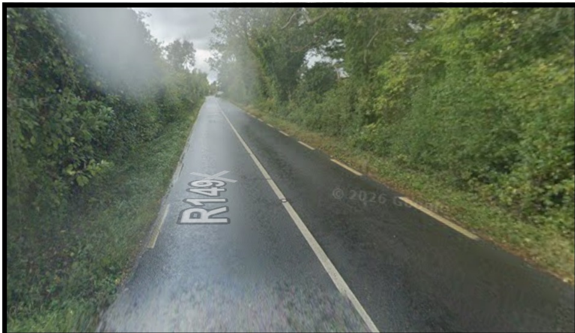
Figure 2.3 – R149, View West at Site
